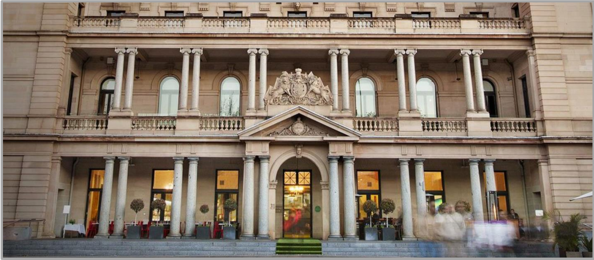
Sydney Customs House, Alfred Street, Circular Quay.
