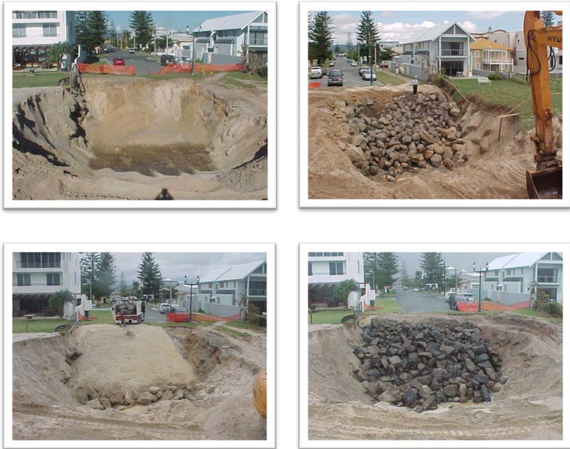
Figure 13 Construction of a seawall on a Palm Beach street end
