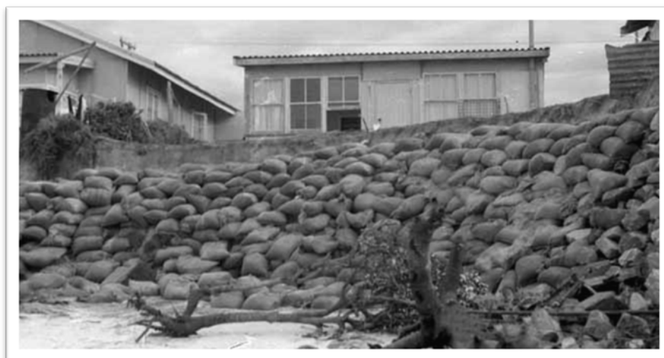
Figure 7 Sandbags used as emergency protection, 1967 storms
