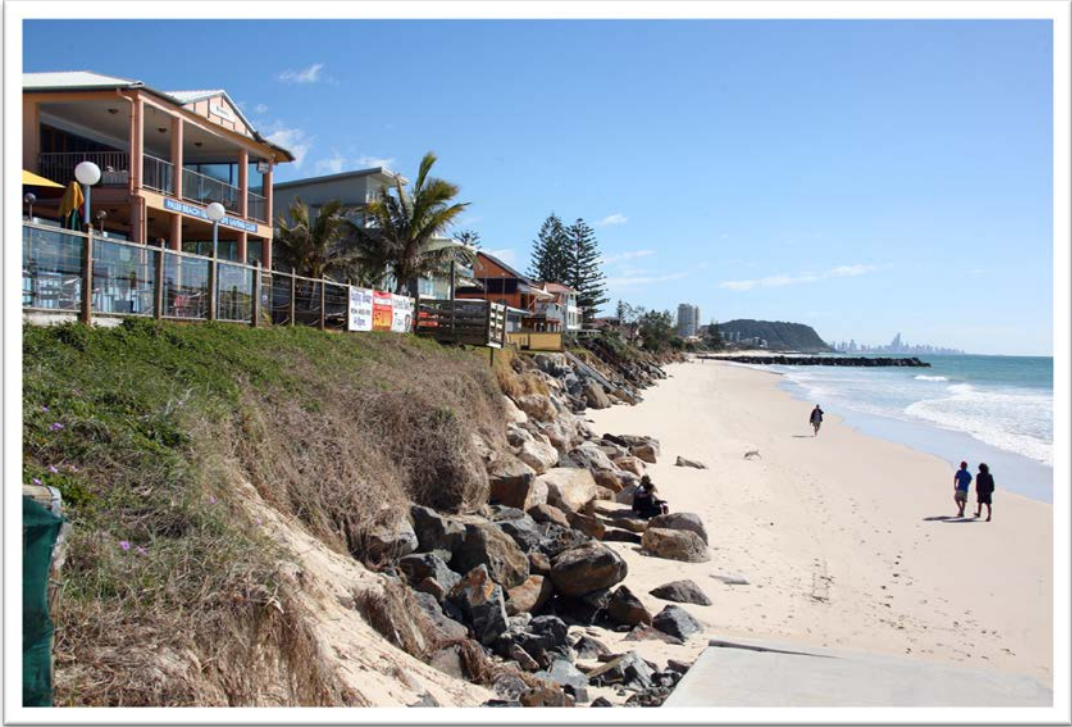
Figure 9 Exposed seawall at Palm Beach, 2012 (Source: GCCM)
