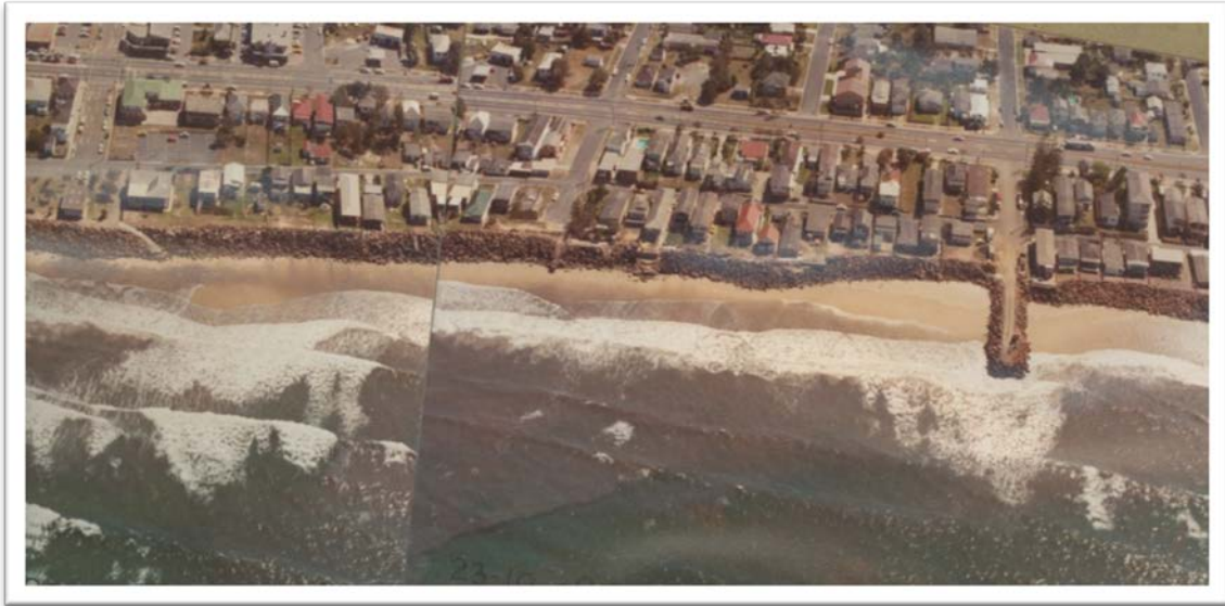
Figure 8 Seawall exposed at Palm Beach, 1989
