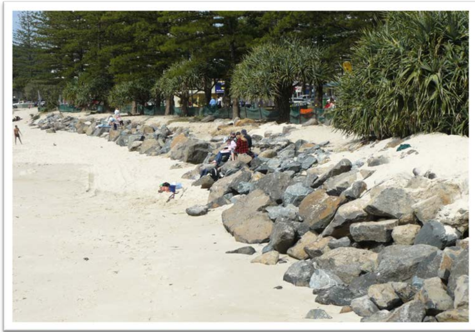
Figure 14 Exposed seawall at Burleigh Beach built to protect the adjacent Justin Park, 2008
