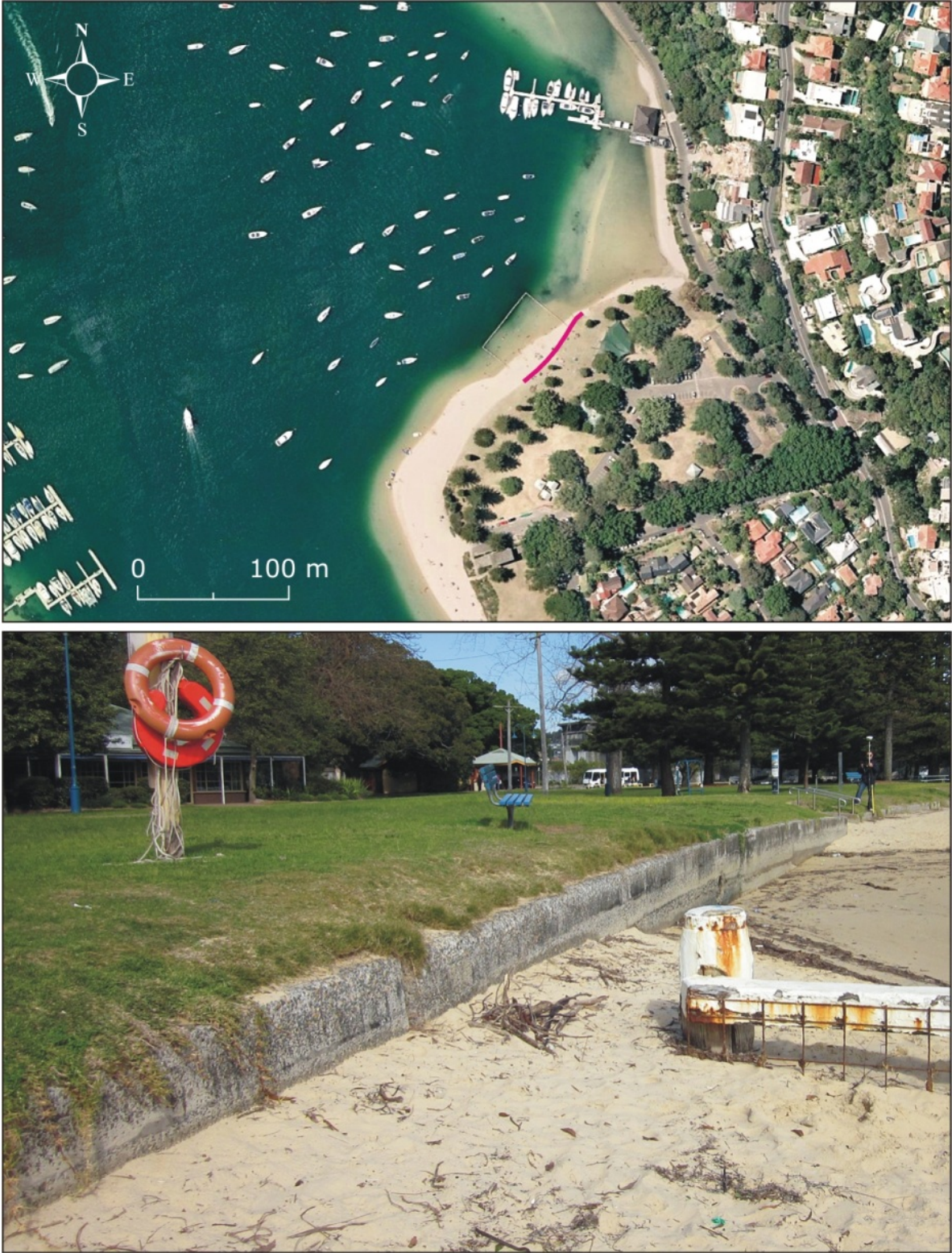
Figure 2.4 Clontarf Seawall 2 at Pool Enclosure 27 July 2001
