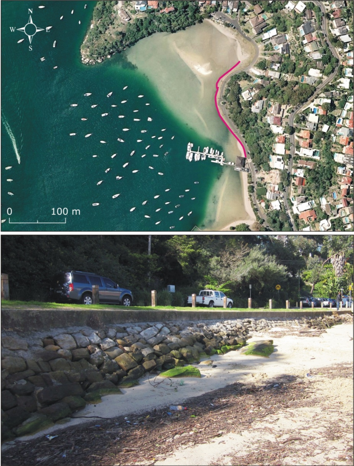
Figure 2.3 Clontarf Seawall 1 Between Sandy Bay and Marina 27 July 2001
