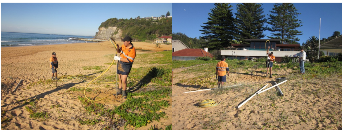
Figure 2.5 Borehole Drilling on the Dune Fronting Number 5 Allen Avenue
