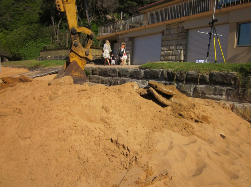
Figure 2.11 Excavation of Seawall Toe Protection Blocks
