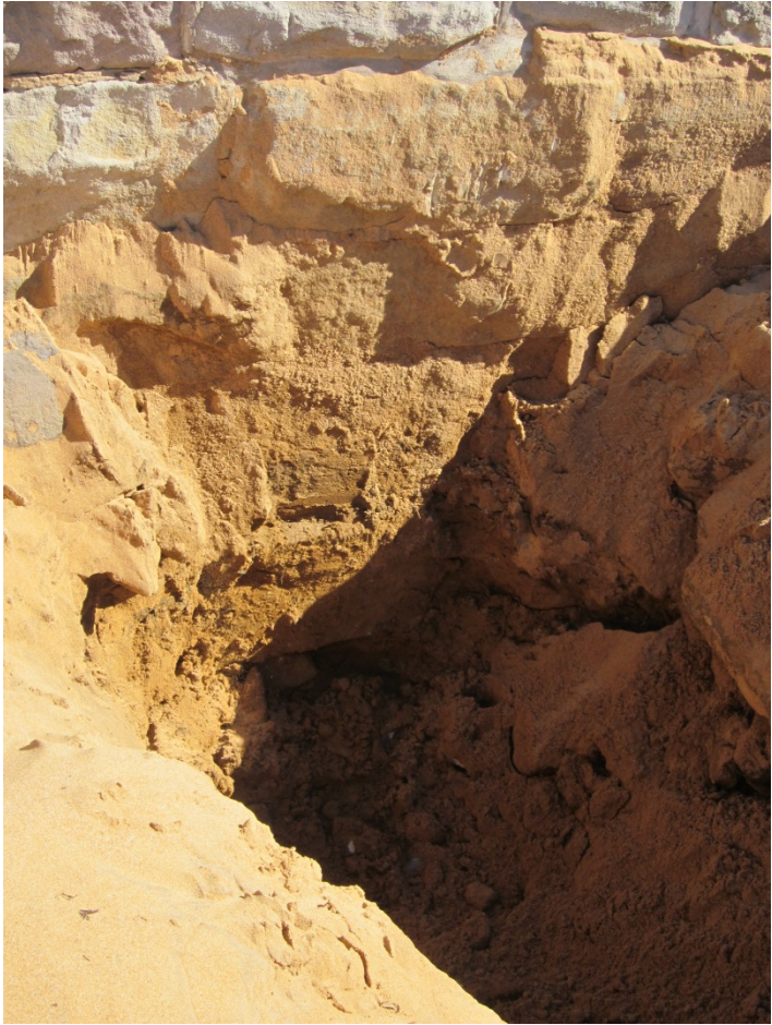
Figure 2.12 Seawall Toe Exposed at Test Pit TP1
