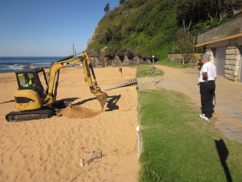
Figure 2.10 Excavation of Test Pit TP1
