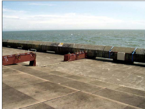
Figure 22 Two overtopping tanks on the crest of vertical seawall
