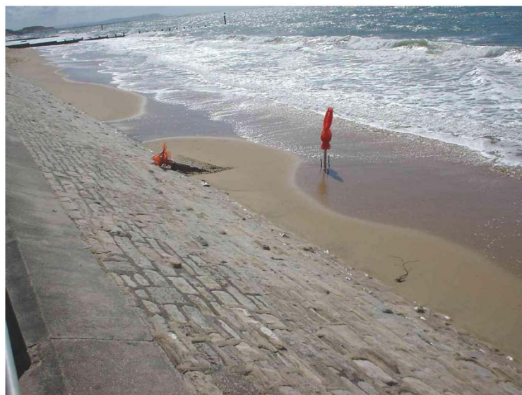
Figure 20 Tell-Tail scour monitors at Southbourne
