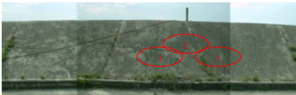
(a) A photograph of the landward side of a seawall
