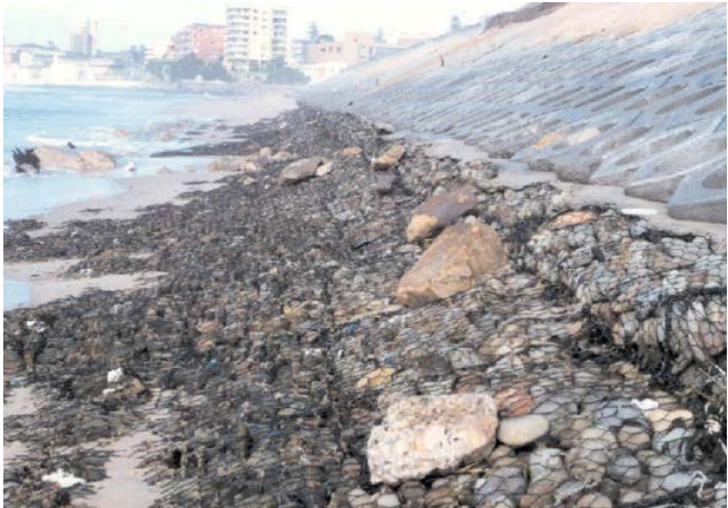
(a) Damaged gabions, Cronulla seawall, 1986
