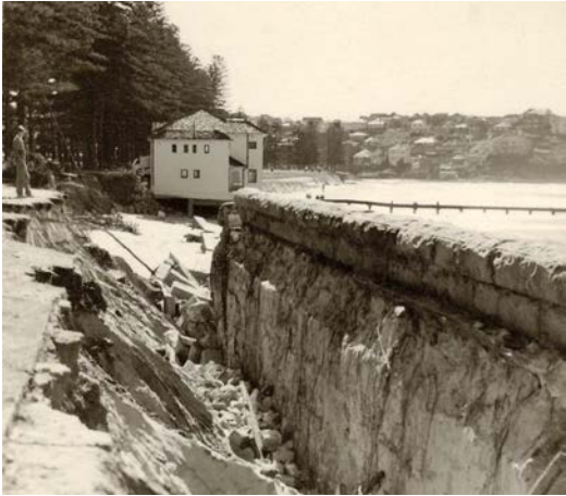
(c) North Steyne collapsed seawall, 1950
