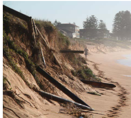
(b) Beach erosion at Narrabeen, 2011
