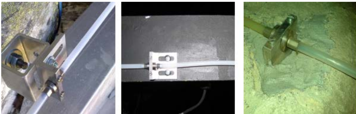
Figure 11 SOFO sensors mounted on different materials
