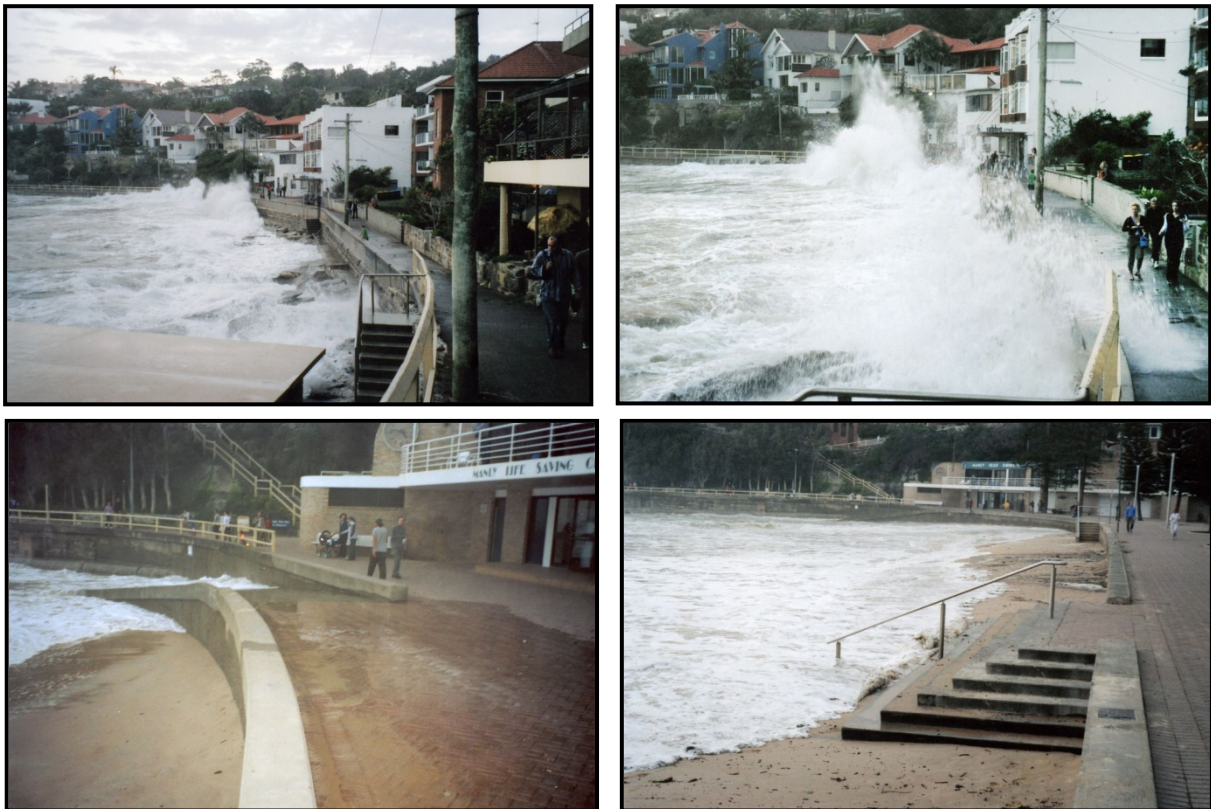
Figure 7 (Top) Wave overtopping the Manly to Shelley seawall; (Bottom) Wave runup at Manly LSSC boat ramp and Manly beach stairs (Victoria Parade)
