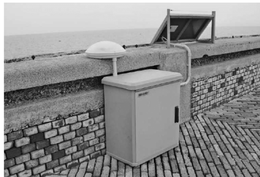
Figure 12 Fully equipped GPS measurement station on the breakwater
