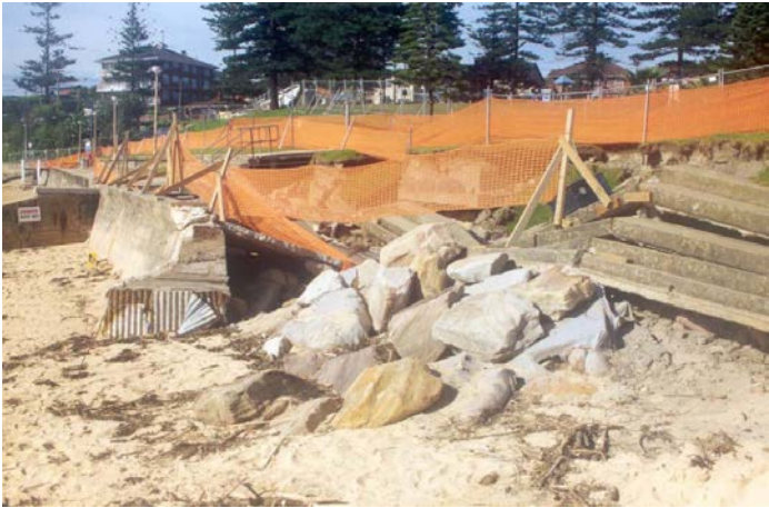
(b) Dee Why collapsed seawall, 1998
