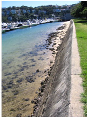
(a) Solid Concrete (Mosman Council)
