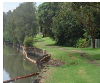
Figure 1 Anchored bulkhead wall – anchor pull-out failure mode
