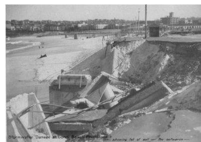
Figure 2 Rigid gravity wall – Rotational slip failure mode
